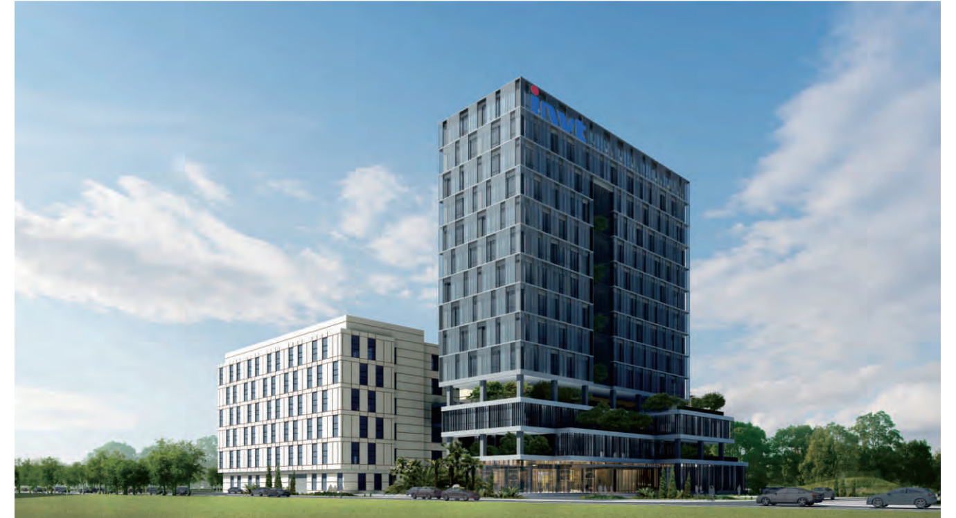
Shenzhen Industrial park
